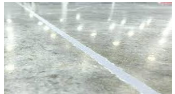
Polished Concrete Floors - Slice through hard Polyurea joint sealant without melting.
