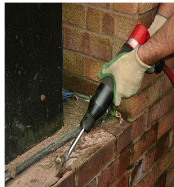
Mortar Removal
