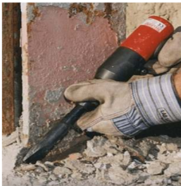
Scraping Iron & Rebar Rods from Concrete
