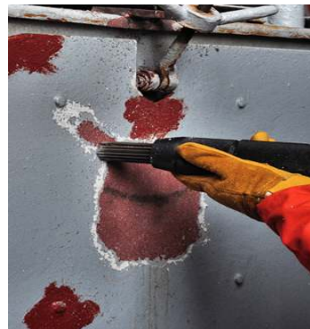
Paint & Coating Removal from Iron, Steel, Thin
