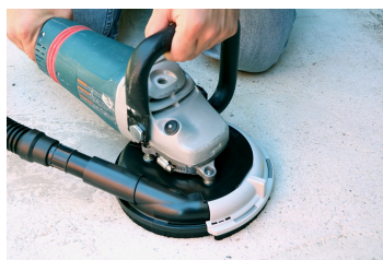
Concrete Surface Grinding
