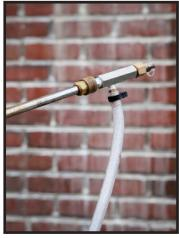
A Contractors applies product with an EC Jet low pressure system using a high volume injector nozzle. This efficient system allows the contractor to apply the chemical and water for rinsing without stopping to switch tools.
