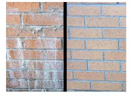
Substrate Cleaned: brick - excess mortar and smears were removed without affecting the mortar joints using NMD 80 and the EC JET.
