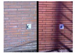
Substrate Cleaned: clay brick - initially cleaned with a competitor's product that left the white haze. NMD 80 removed the residual haze and provided the successful post construction cleaning.
